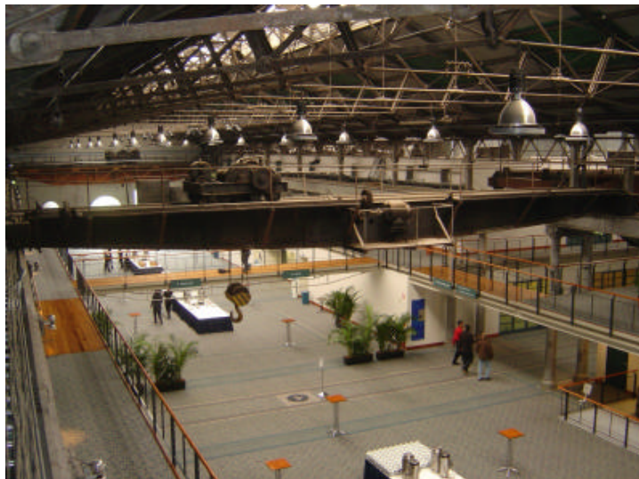
Figure 2. Looking down into the Atrium showing the new structure within the original structure.
